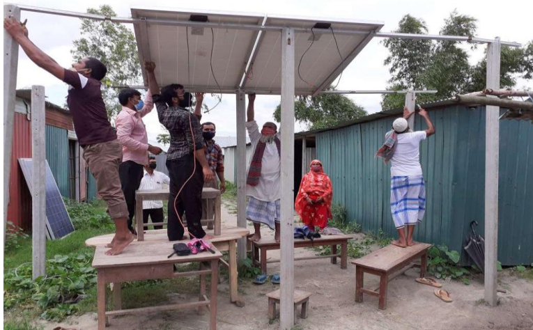
Solar panels dismantled by Para-Solar Technicians before the floods
